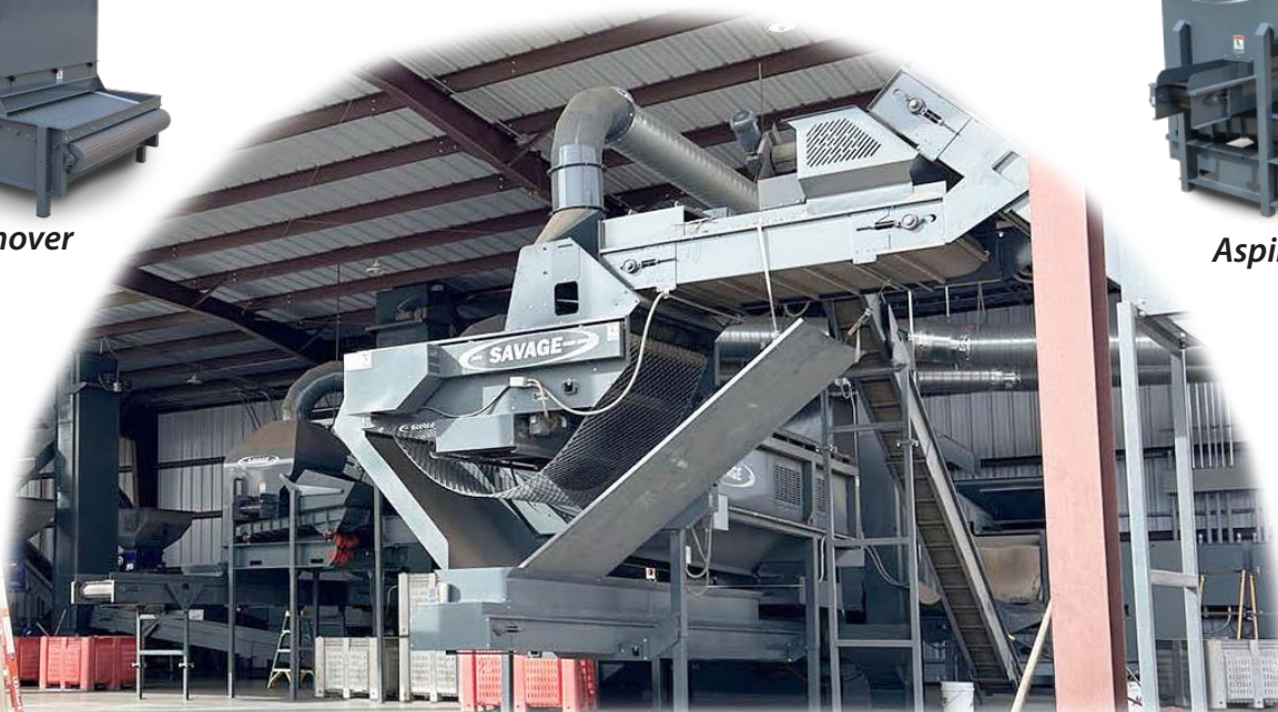
Portion of the Barker Produce/Pure Nuts Cleaning Plant in Las Cruces, New Mexico
